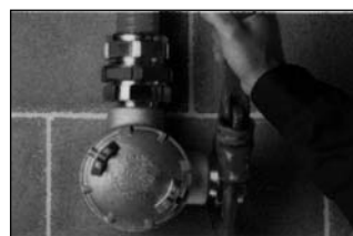
5. Install hub on enclosure
